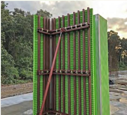
▲ Image shown a set of complete assembled Plasform Panels with double bracing on positioning for casting of a multi-directional wall.
